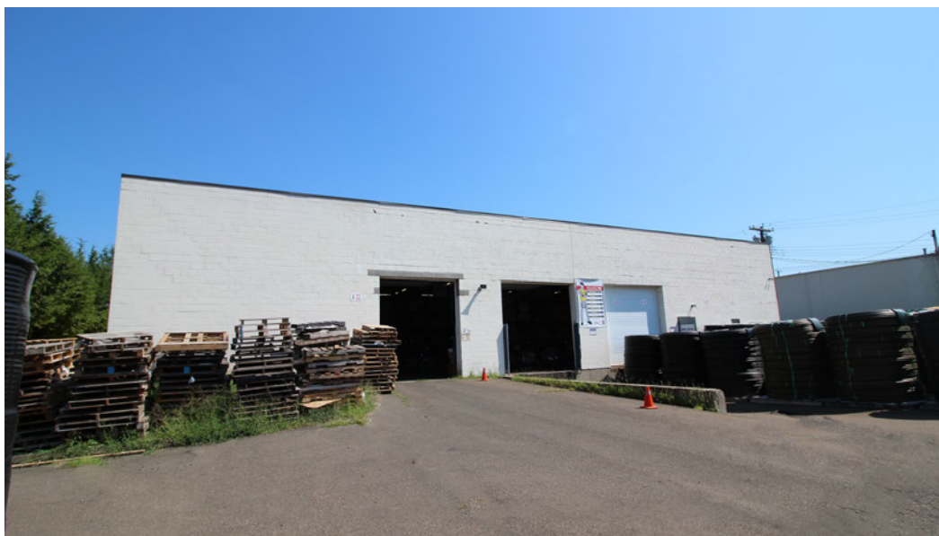
1 DRIVE-IN DOOR & 2 LOADING DOCKS
