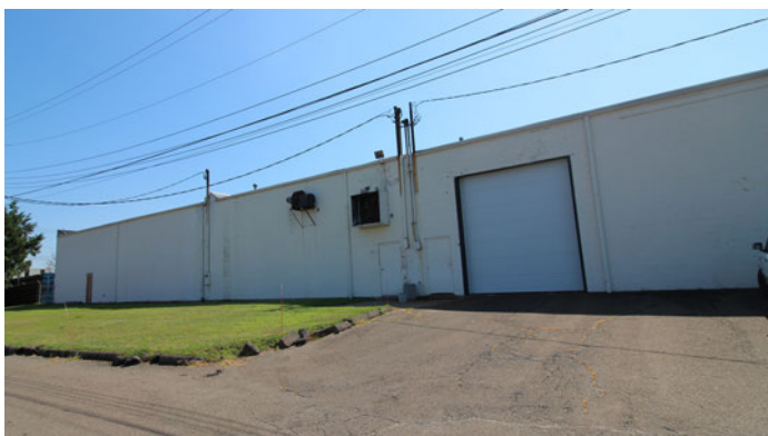
FIVE DRIVE-IN DOORS WITH DRIVE-THRU CAPABILITY
